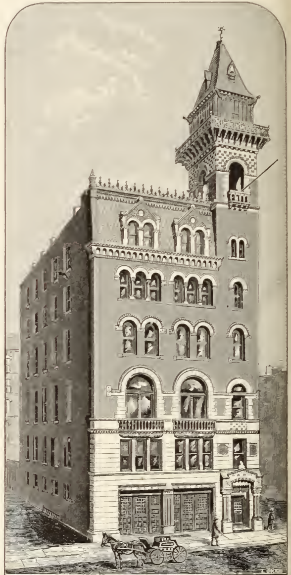
NEW FIRE HEADQUARTERS. [Otis Brothers' Elevator.]
