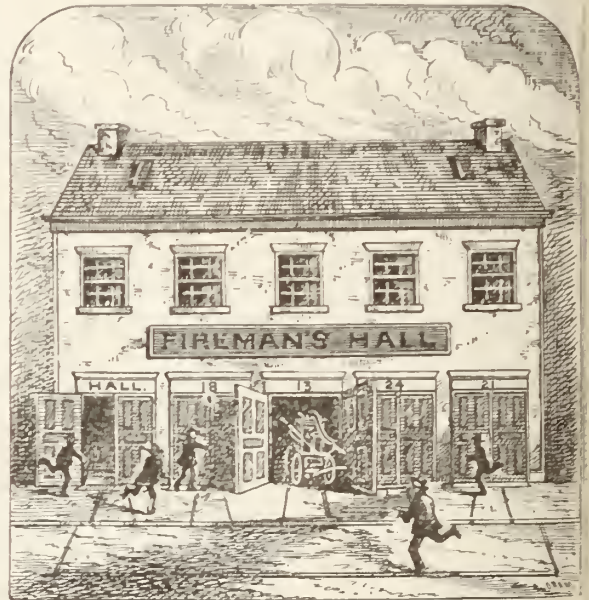
FIRST FIREMEN'S HALL.
