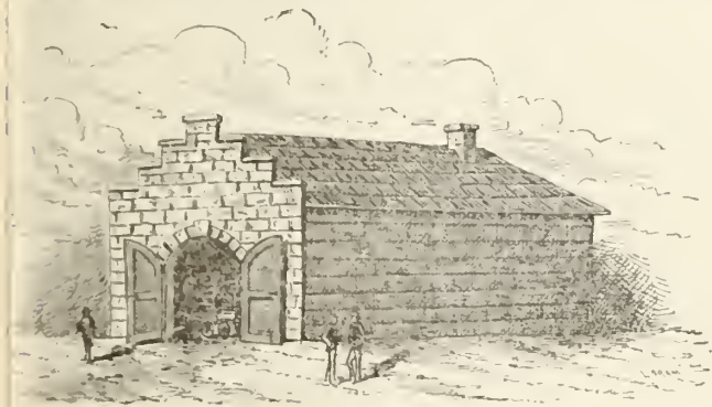
OLD ENGINE HOUSE, HANOVER SQUARE.
