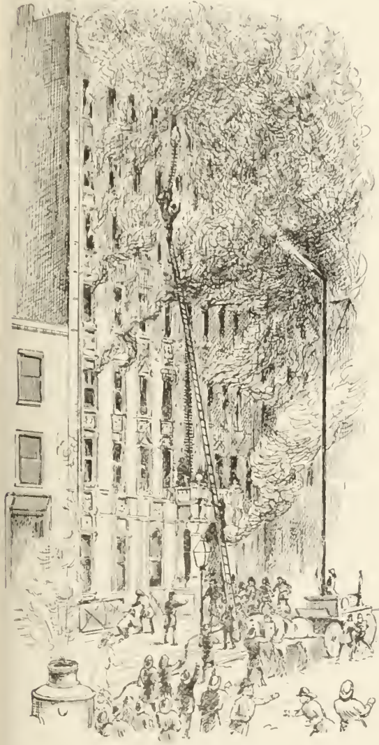
BURNING OF ST. GEORGE FLATS.
