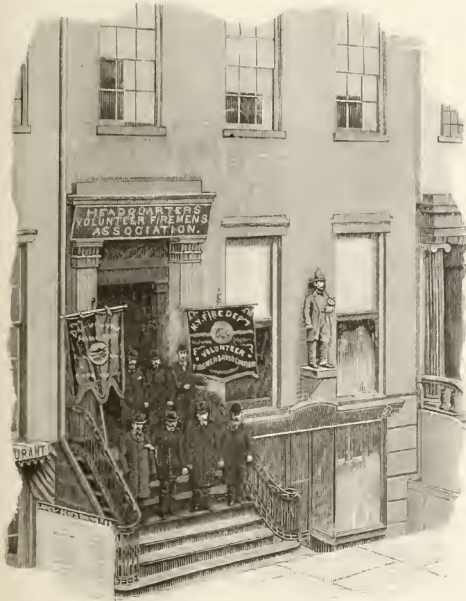
HEADQUARTERS OF VOLUNTEER FIREMEN'S ASSOCIATION. [143 Eighth Street.]
