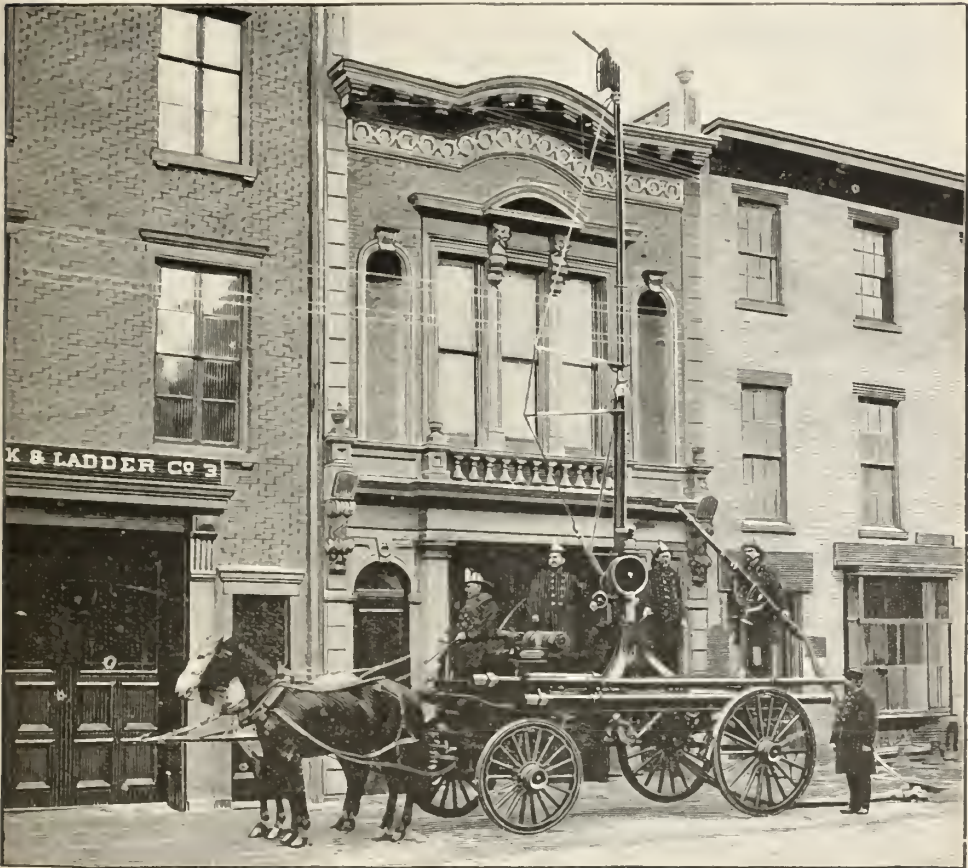
WATER TOWER EXTENDED.
