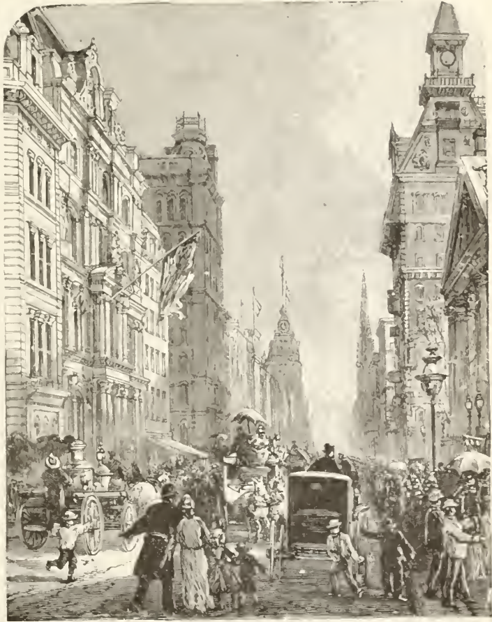
BROADWAY, SOUTH OF VESEY STREET.
